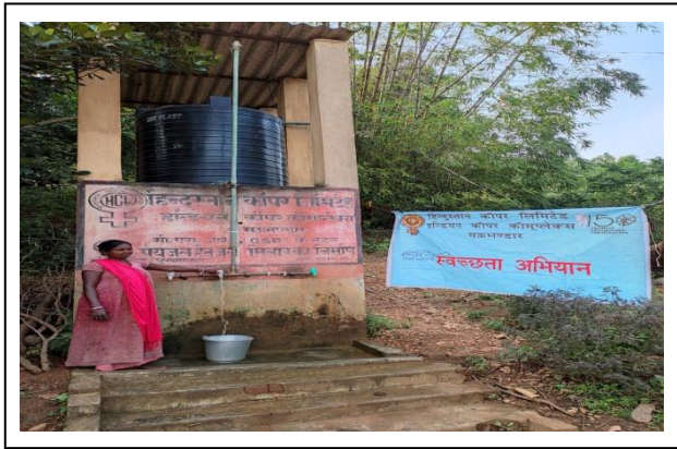
Repair of existing Jal Minar at Kendadih Village near ICC Unit
