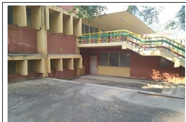
After Cleanliness Drive – Several places in Plant Area of KCC Unit
