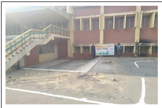
Before Cleanliness Drive – Several places in Plant Area of KCC Unit
